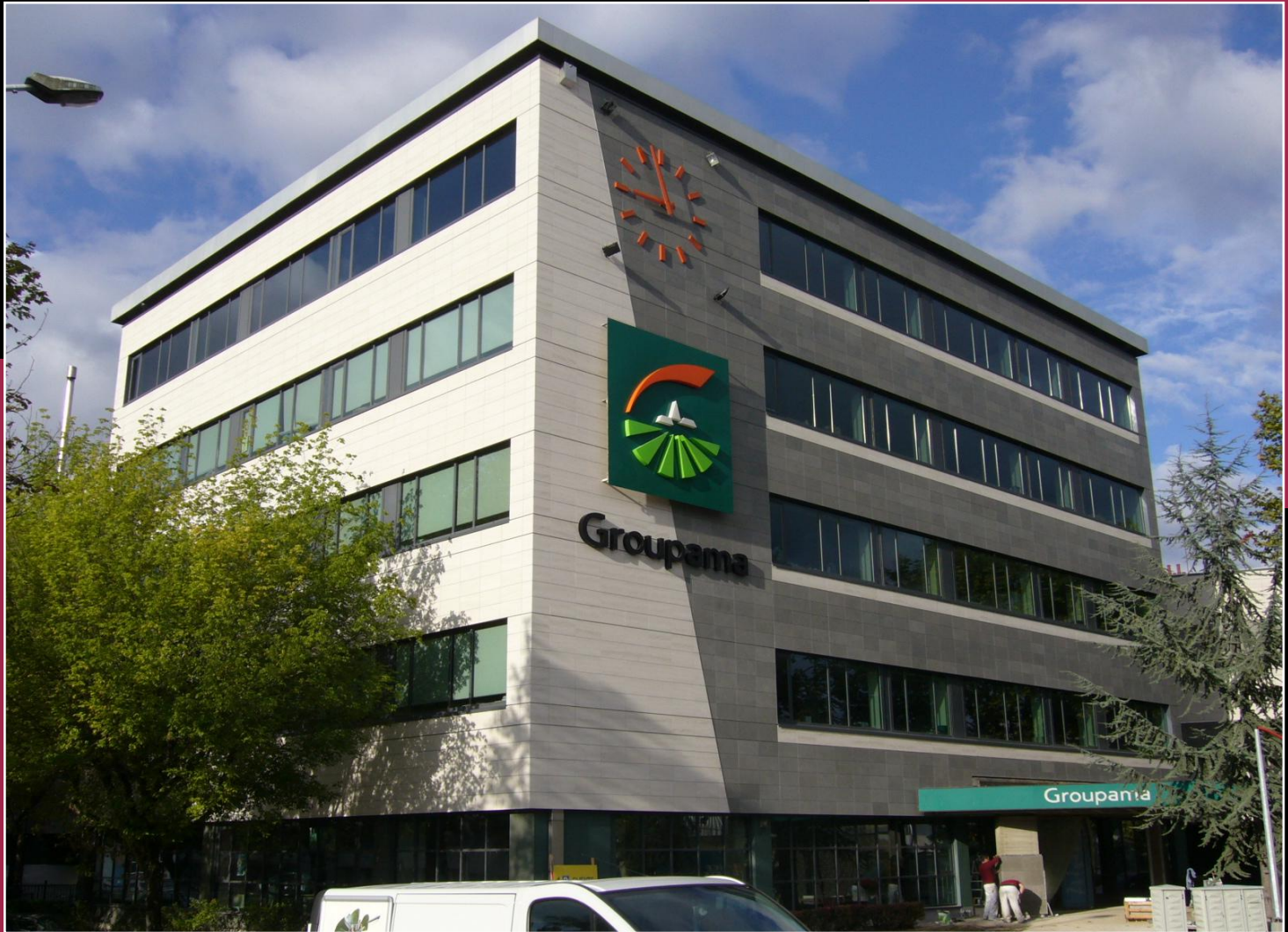
Groupama building, France (2010). Stone: Semi-Rijo LR and Valverde honed. Édifice Groupama, France (2010). Pierre: Semi-Rijo LR et Valverde adouci.
